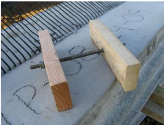
Figure 7 – Diagonal clamp
