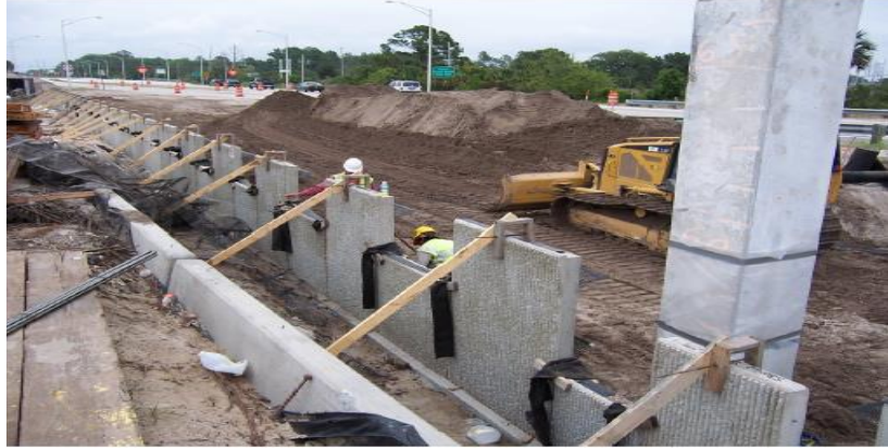
Figure 6 – Header clamp and brace in position on full panels
