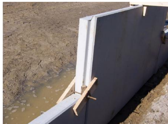
Figure 8 – Diagonal clamp used to hold the panel in place
