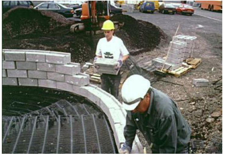
Figure 5 Geogrid overlaps on the inside of curved walls
