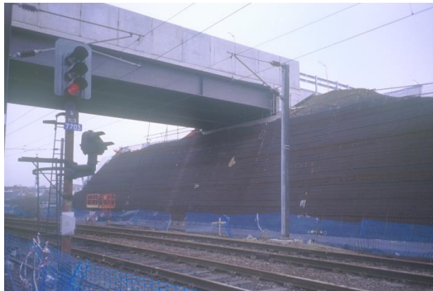
Figure 1 TensarTech TR2 temporary bridge abutment
