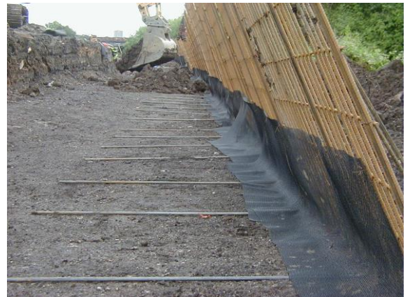
Figure 2 – L bars and face units in place
