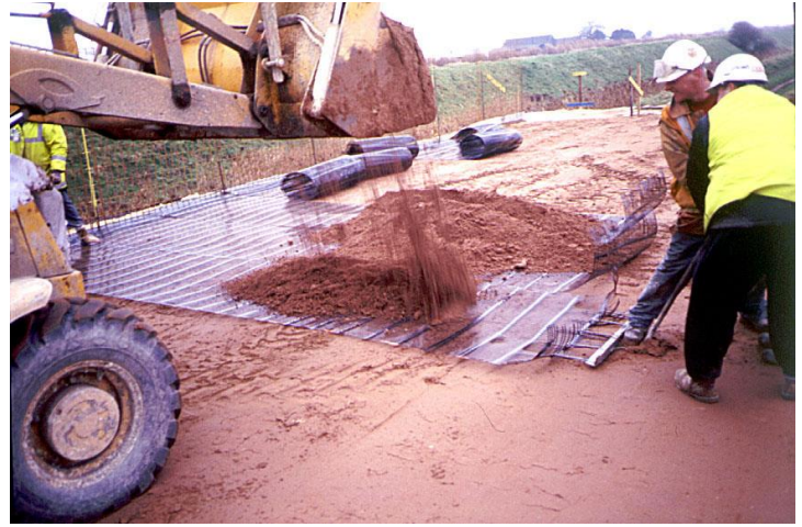
Figure 5 – Tension the geogrid and placing the fill
